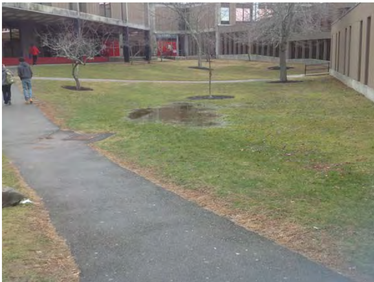
Figure 1: View of B.M.C. Durfee High School main entrance that faces Elsbree Street. The image captures the variances in gradient with the catch basin not fully utilized as standing water is visible within two to three feet of the drain (Photo taken January 26, 2017).
