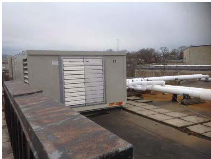
Figure 12: Mammoth Inc. HVAC units on the roof of the high school building. The current piping system once contained glycol, but now utilizes water. Due to cycling up in concentration, frequent corrosion issues occur due to lack of corrosion control measures of the City water entering the system (Photo taken January 26, 2017).
