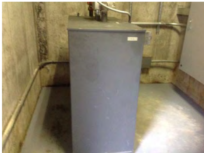
Figure 8: Two elevators were on site. This elevator machine room was at the main entrance of the building. No visible hydraulic fluid in the room or evidence of spills in either machine room was observed (Photo taken January 26, 2017).
