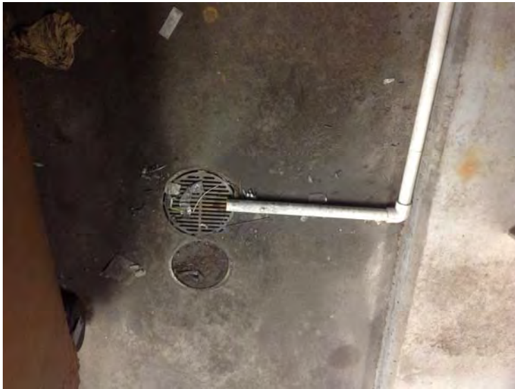
Figure 5: Drainage in the same room as Figure 4, which leads to the City's drainage and combined sewer (Photo taken January 26, 2017).
