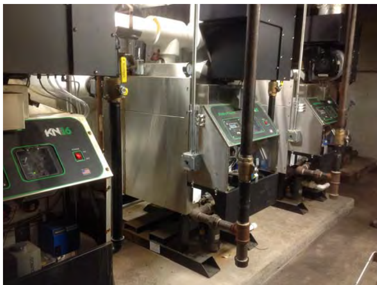
Figure 4: Three remaining boilers that supply the Buildings 1-3. These boilers are relatively new and were installed three years ago and are maintained and monitored by ENE Systems Inc. based out of Canton, MA (Photo taken January 26, 2017).
