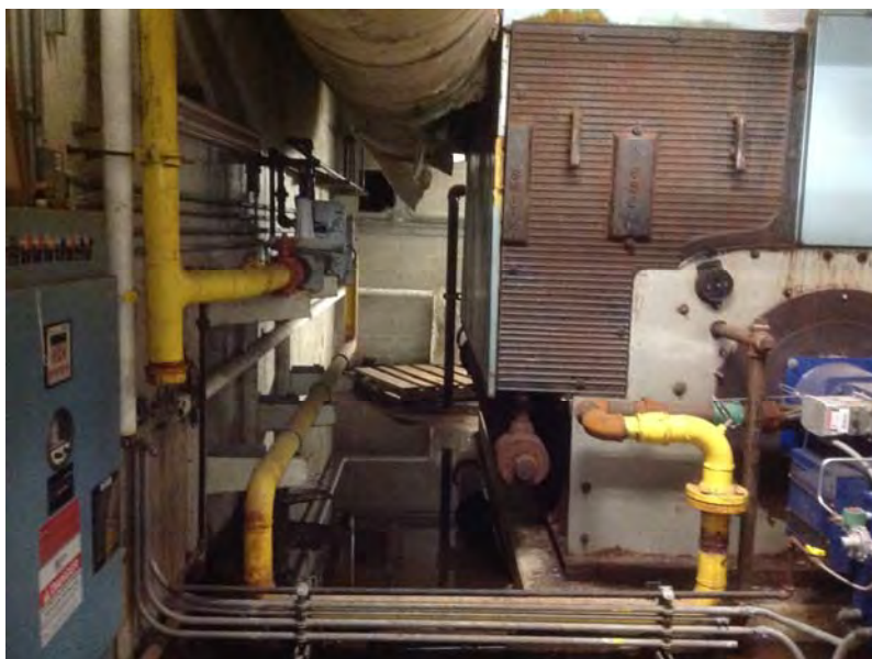
Figure 2: View of the two boilers underneath the swimming pool that supply Building 4. Due to the pressure release valve, water vapor is typically discharged into this room and can be identified by the standing water on the floor, no drainage was visible (Photo taken January 26, 2017).
