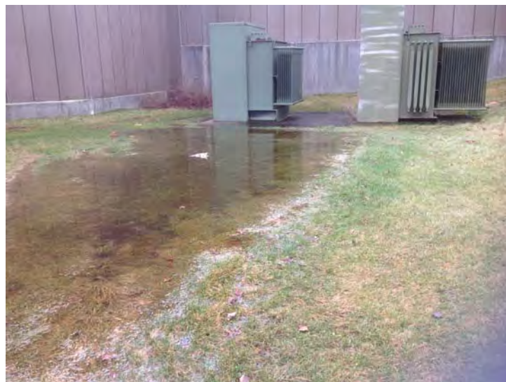
Figure 10: Two of four transformers on Site. Due to the gradient both transformers reside in low-lying areas with poor drainage (Photo taken January 26, 2017).
