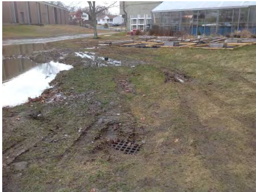
Figure 6: Changes in gradient on the property created areas of saturated soil with poor drainage. In this instance the standing water was in the proximity of two drains but was unable to capture the runoff (Photo taken January 26, 2017).
